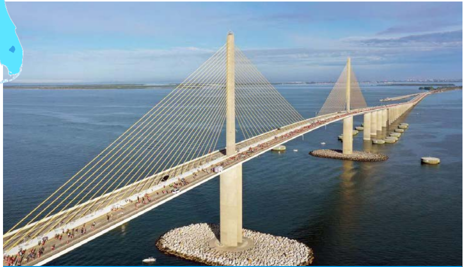
Tampa Bay's Sunshine Skyway Bridge connects southern Pinellas and Manatee counties
