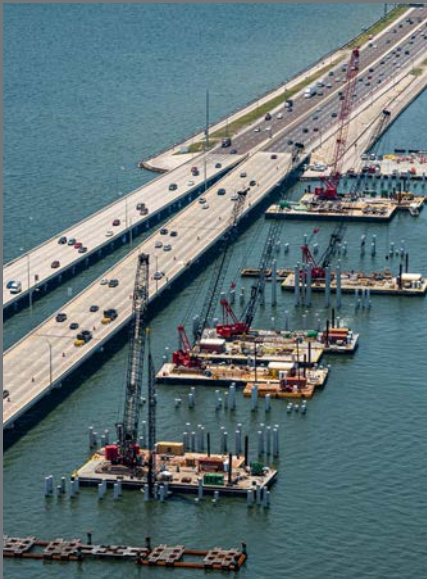
The new 8-lane Howard Frankland Bridge under construction in Tampa Bay.
