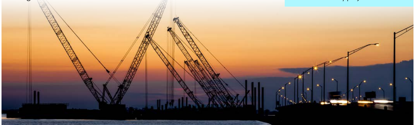
Construction on Tampa Bay's new Howard Frankland Bridge
