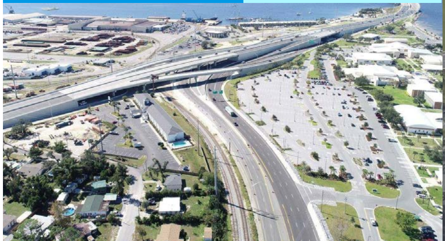
23rd Street Flyover
