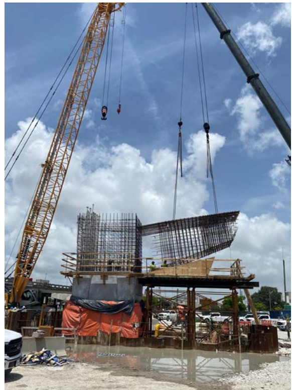
I-395 Pier Construction
