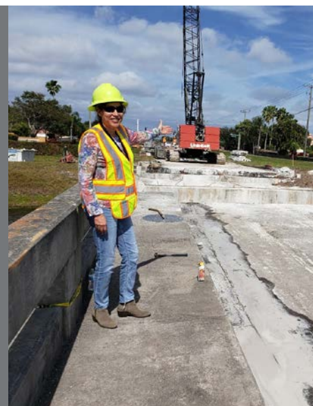
El Clair Ranch Road Bridge Replacement Project in Palm Beach County
