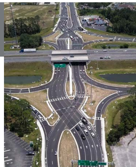
Northeast Florida's first diverging diamond interchange at I-95 and S.R. 200/A1A
