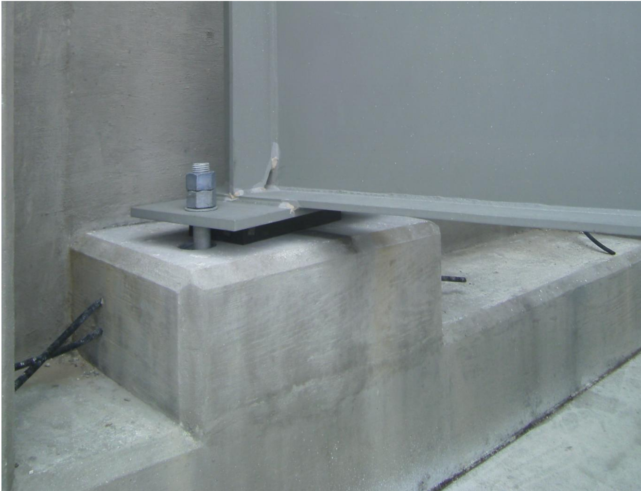
Typical Neoprene Bearing Pad with Formed Bolt Holes (note the grout tubes protruding from the pedestal)
