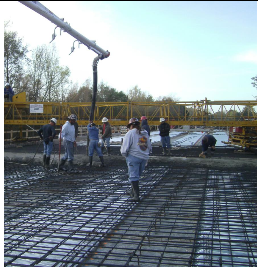
Deck Placement Using a Concrete Pump
