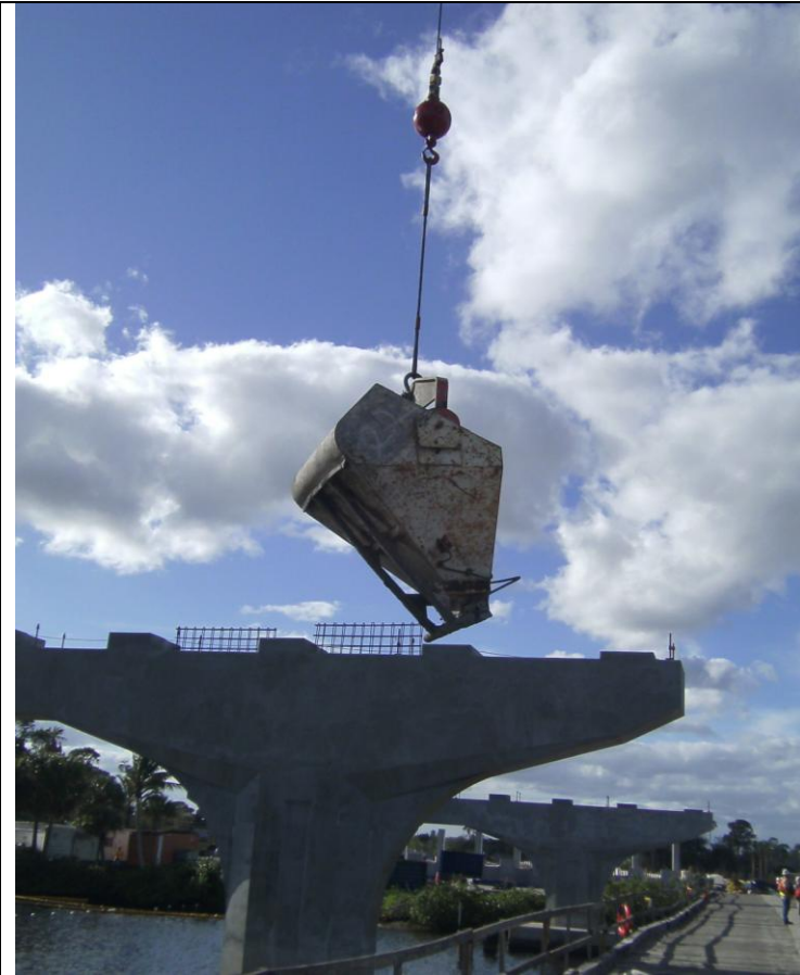
Concrete Placement Bucket
