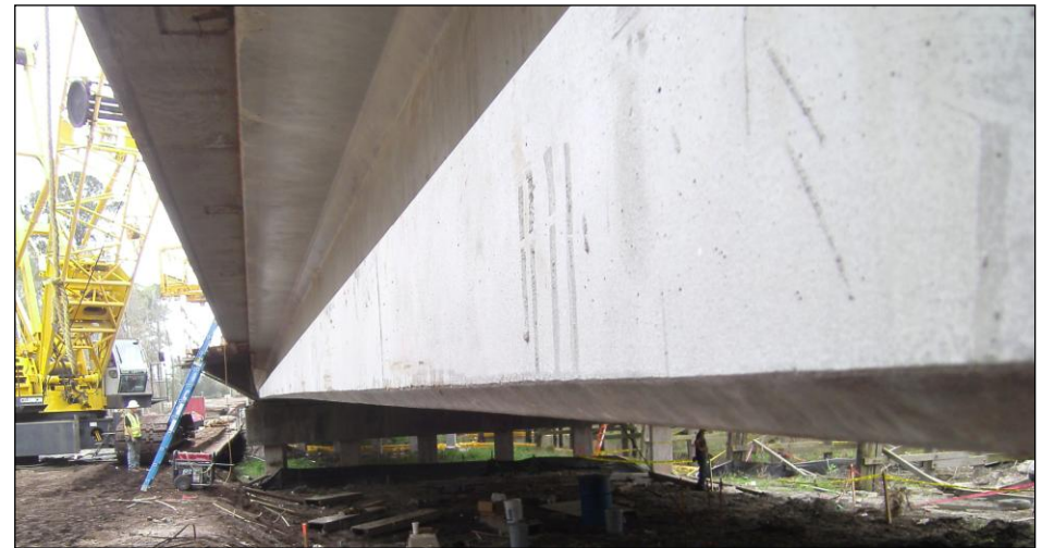
Pictured to the right, is a similar girder to the one above after deck casting – notice the relatively flat profile of the girder that has resulted because of the downward deflection caused by the deck load thus reducing the camber
