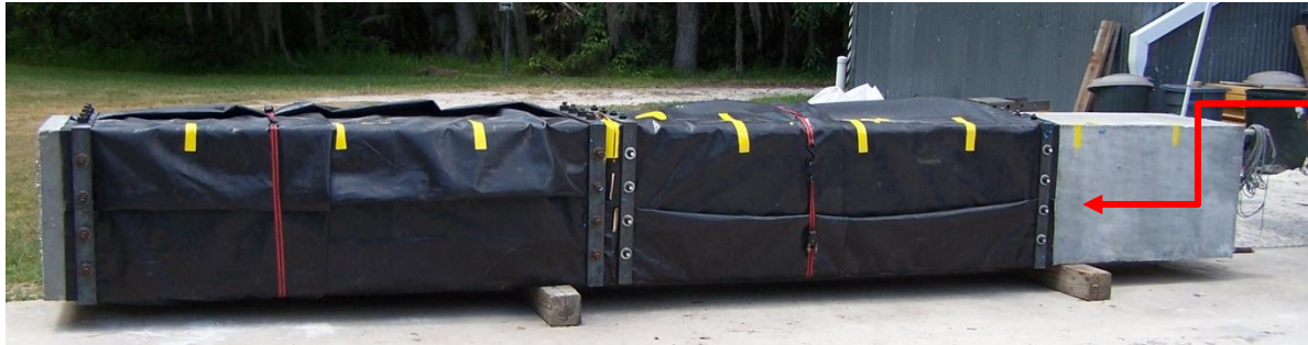
Attaching Grout Membrane
