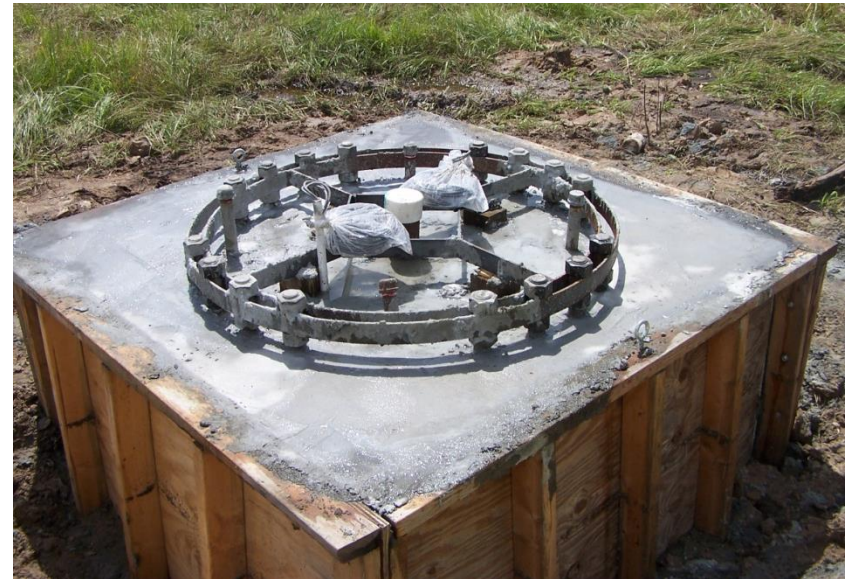
Cast-in Place Cap
