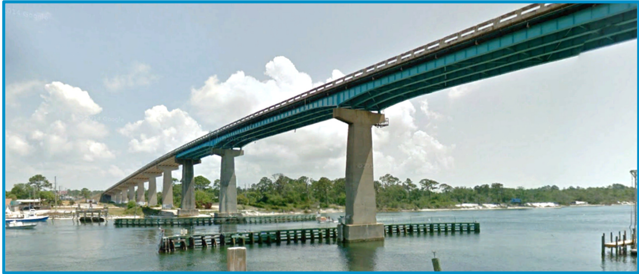
Source: "Perdido Key Bridge." 30°18'44.27" N and 87°25'36.41" W. Google Street View. Image capture May 2011.
