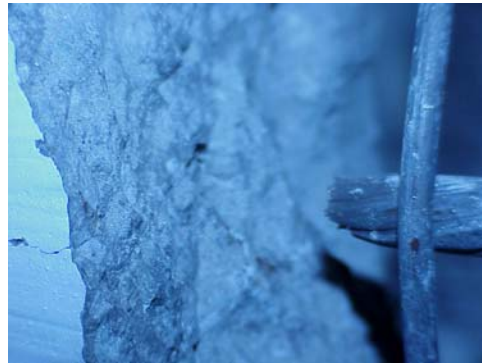
Figure 17 – Ruptured Bar
