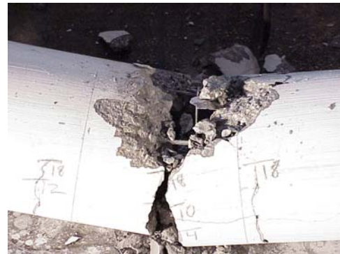
Figure 13 – Specimen After Failure
