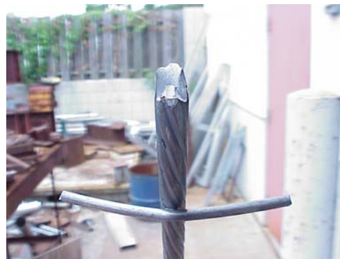
Figure 8 – Fracture Through Weld With Spiral Reinforcement Shown
