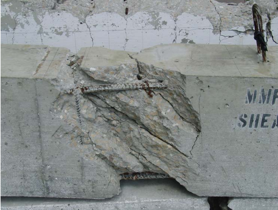
Fig. 11 MMFX Test 4 Beam
