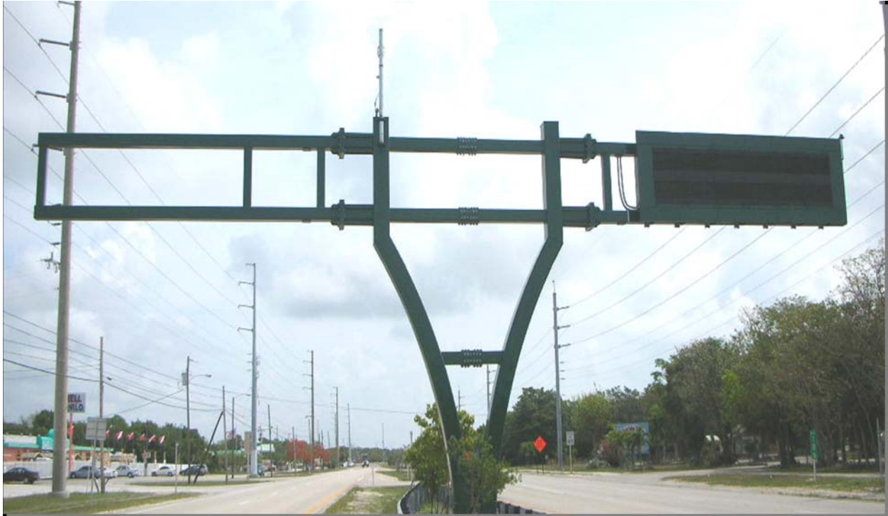
Figure A.6 – FDOT District 6 DMS Structure
