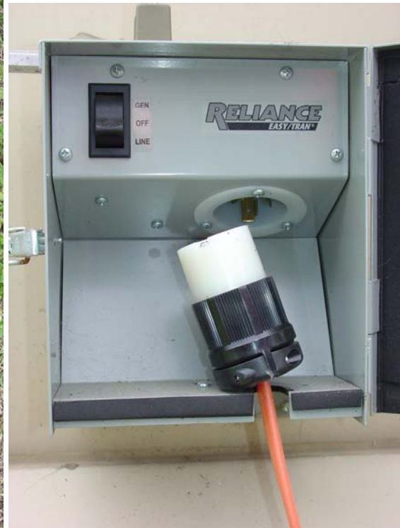
Generator Cable Twist Lock Connector can be secured to transfer switch with pad lock.
