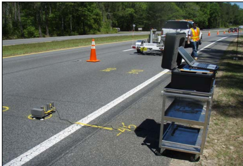
Figure 3.1. Field Test Set-Up.
