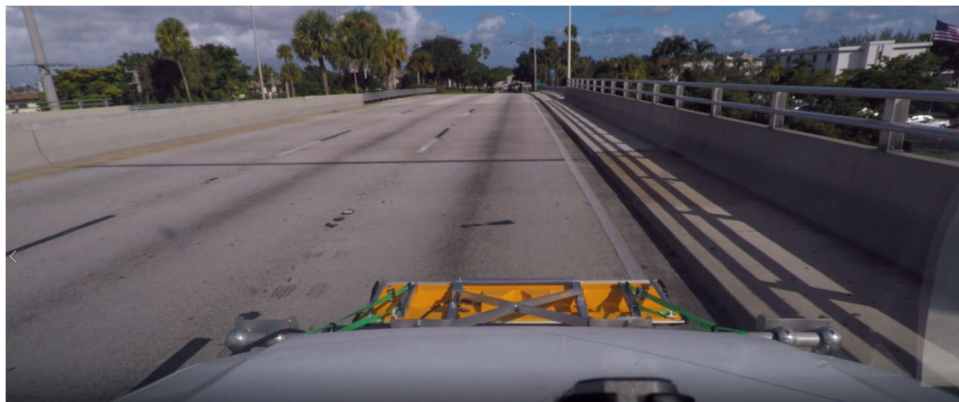
Figure 16: General view of Broward bridge deck. Eastbound lane, right side. Camera pointing east.
