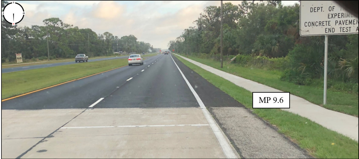
Figure 13: Transition from south end of the test section to the regular roadway on SR 5 in proximity of MP 9.6.
