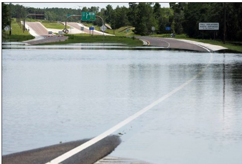
Figure 1. Flooding at Suncoast Parkway in Hernando County, FL (courtesy: Tampa Bay Times/Will Vragovic ).
