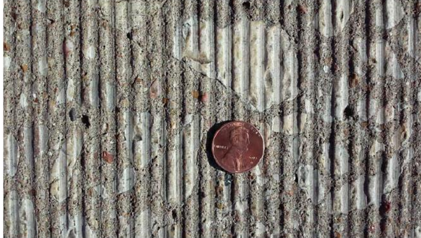
Figure 31. Diamond-ground surface in Texas (Smit et al., 2016)
