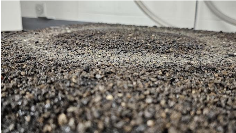
Figure 42: Roughness of the Bauxite HFCS Slab
