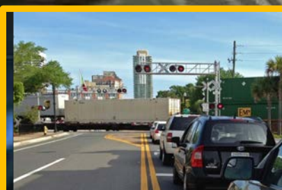
Rail Crossing Notification Systems
