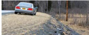
Shoulder is provided along roadway curve.
