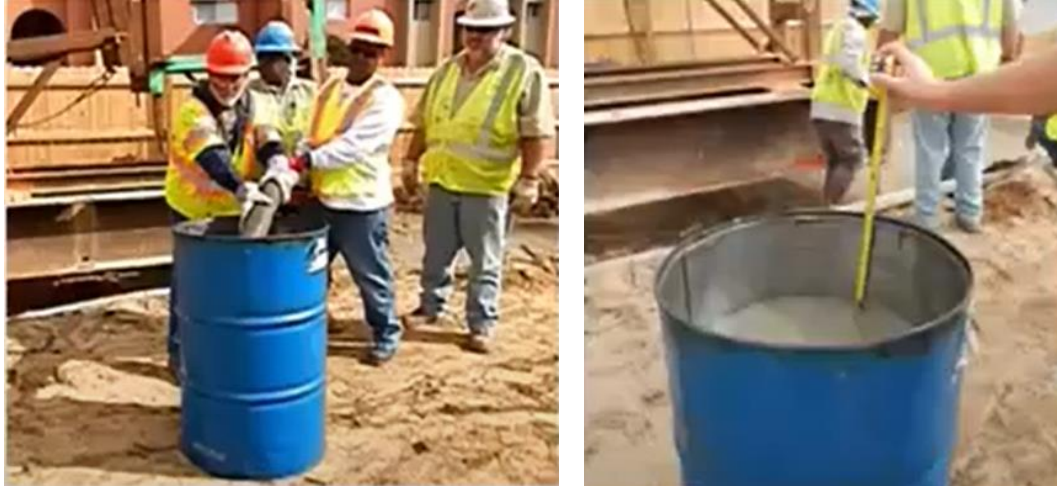
Figure 1.6 Grout pump calibration using 55-gallon drum (Castellanos, 2015)
