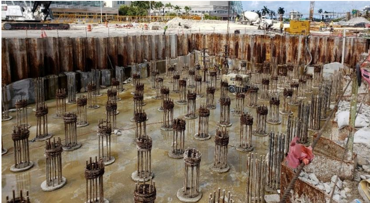
Figure 2.17 I-395 signature bridge center pier construction
