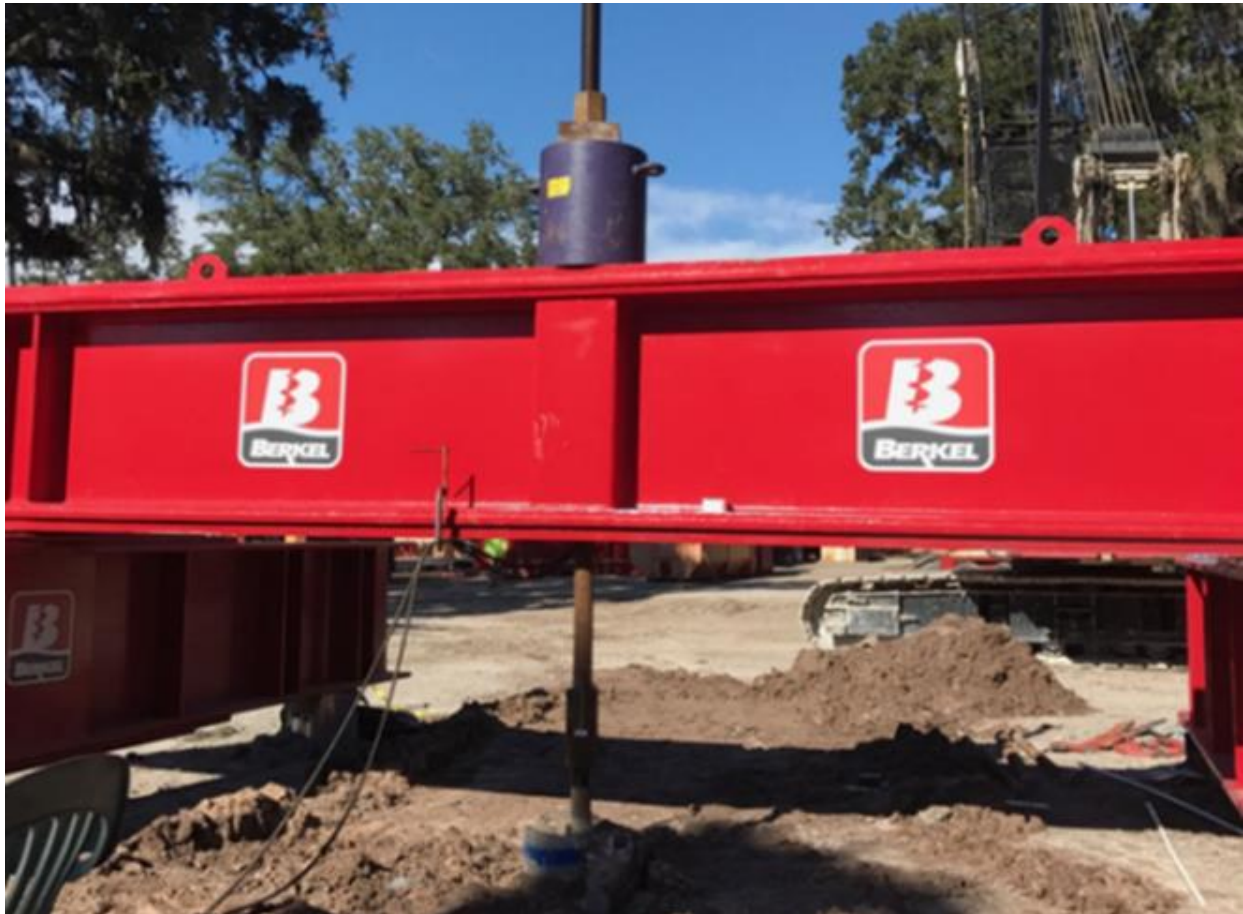
Figure 2.12 Tension load test setup used to extract auger cast pile E-1 (Marinucci & NeSmith., 2017)
