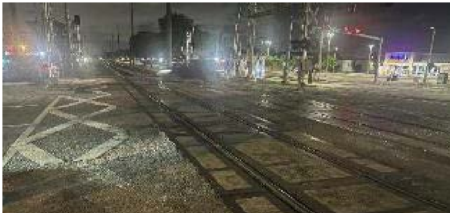
Figure 6-27. Visibility of RDE Pavement Markings at Night at SR-822 @ Dixie Hwy, District 4
