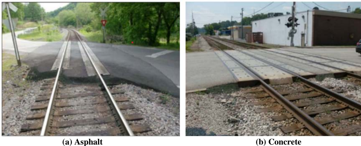
Figure 2-7. Paved Crossing Track Beds and Surfaces (44)
