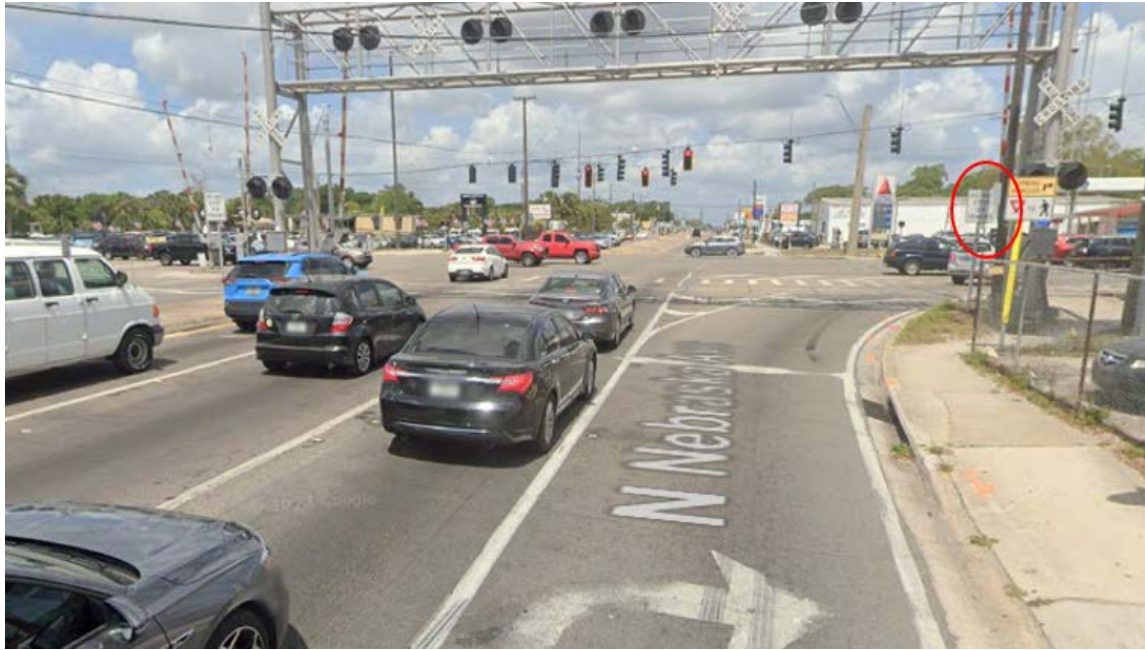
Figure 6-38. Drivers' View When Approaching the Crossing at E Busch Blvd @ N Nebraska Ave, District 7
