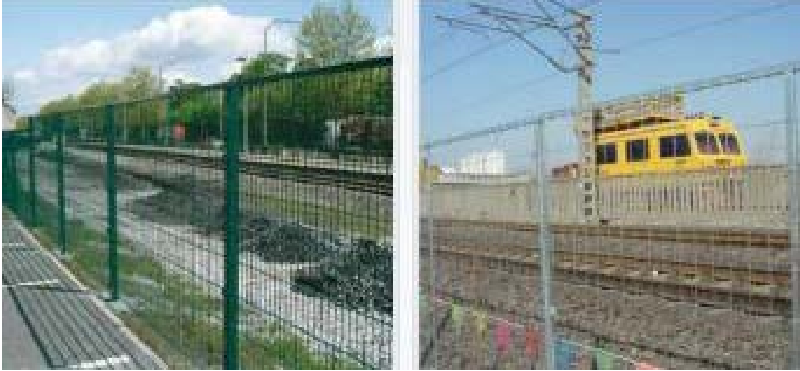
Figure 5-6. Fencing along Railroad Tracks to Deter Trespassing (Source: https://www.steelpalisade.net/palisadefence/railwayfence.html )
