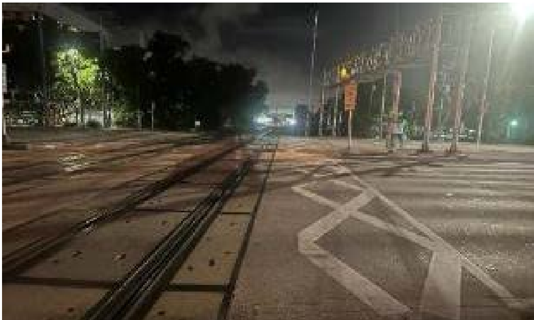
Figure 6-23. Night Visibility of RDE Pavement Markings at W Cypress Creek Rd @ N Andrews Ave, District 4
