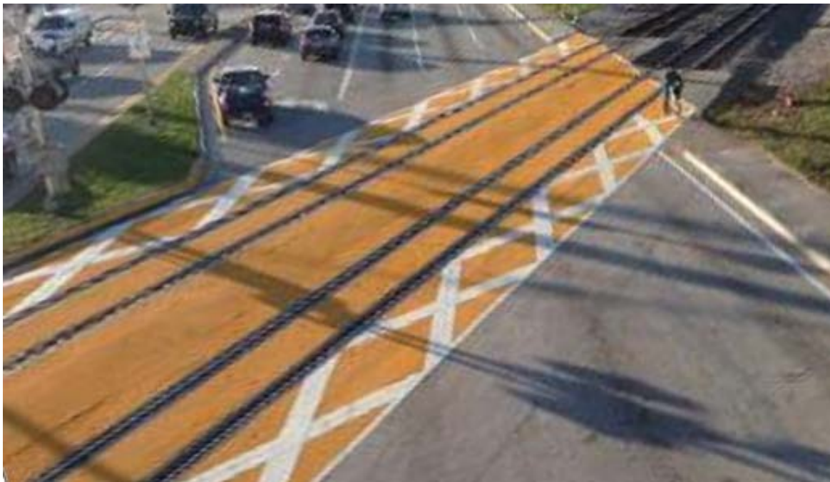
Figure 5-3. RDE on Yellow Pavement Marking Installed in District 4
