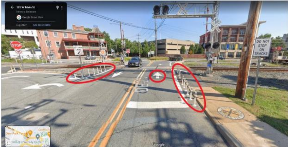
Figure 5-12. Delineators and Pavement Arrows on Eastbound at an HRGC in Newark
