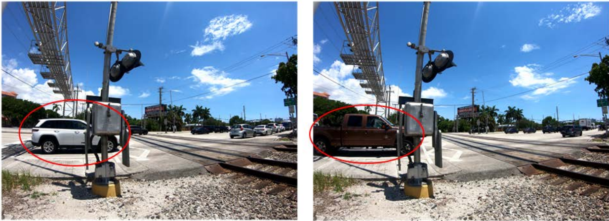
Figure 6-21. Stopping in Zone 2 in Queues on WB at W Cypress Creek Rd @ N Andrews Ave, District 4
