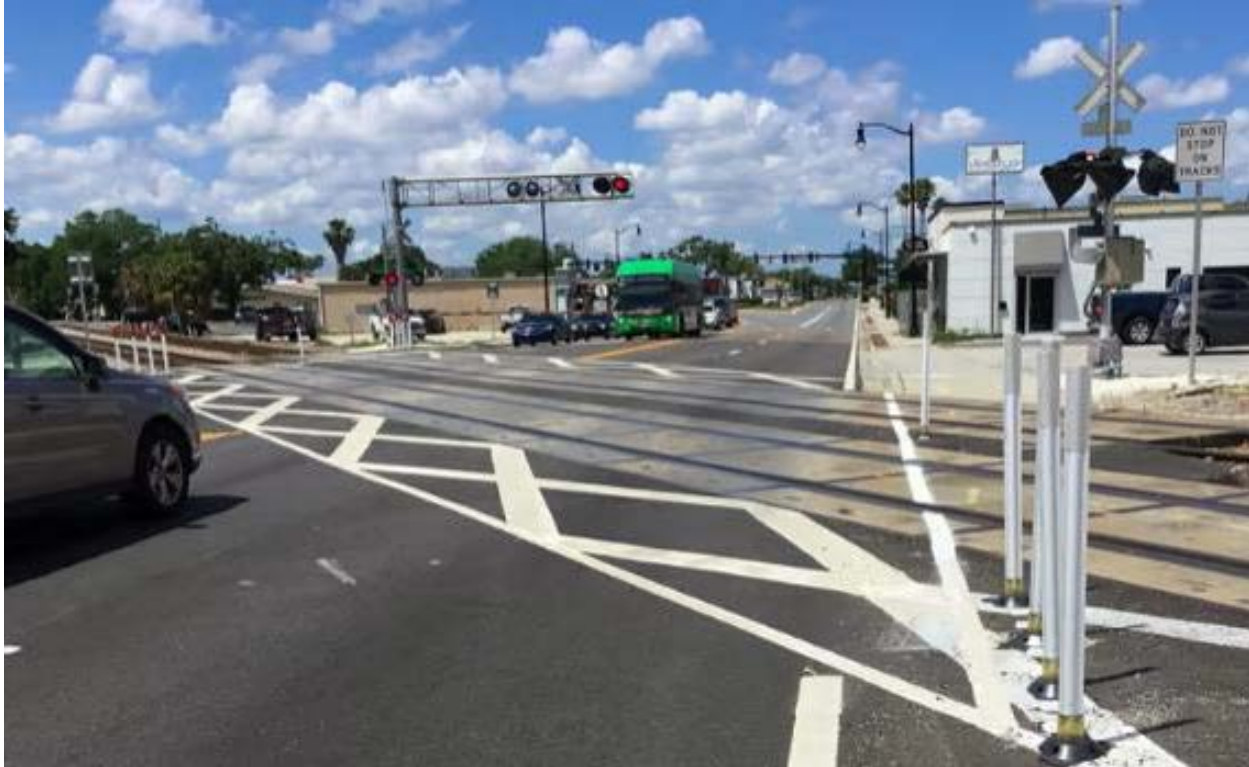
Figure 5-5. Delineators next to Railroad Tracks (Source: https://www.news4jax.com )
