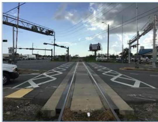
R/R Crossing Looking East
