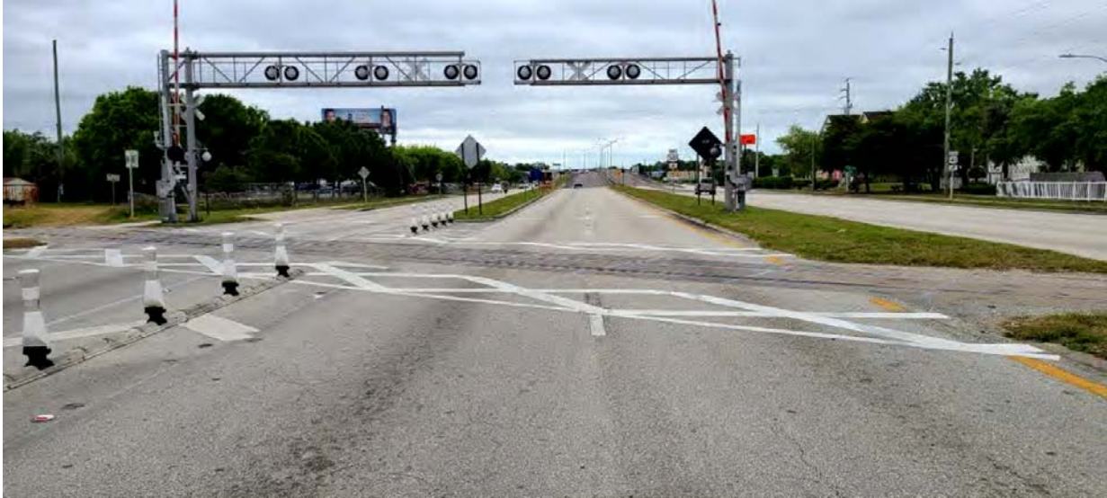
Figure 3-3. Example of RDE Implementation in FDOT District 1 (U.S. 41/301 @ 13th Avenue E)
