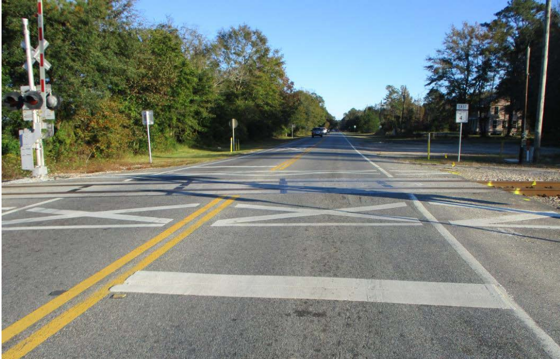
Figure 3-5. Example of RDE Implementation in FDOT District 3 (SR-4 @ SR-95 [US-29] in Escambia County)
