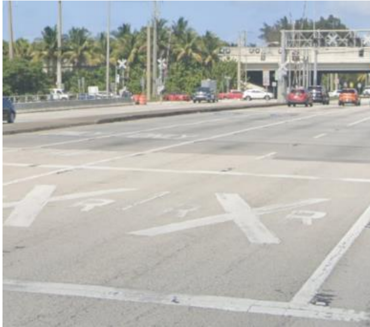
Figure 2-2. Pavement Marking Upstream of a Railroad Crossing (Source: Google Maps)
