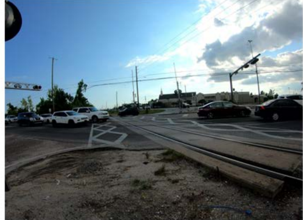
Stopped Vehicles Occupied RDE Pavement Parkings
