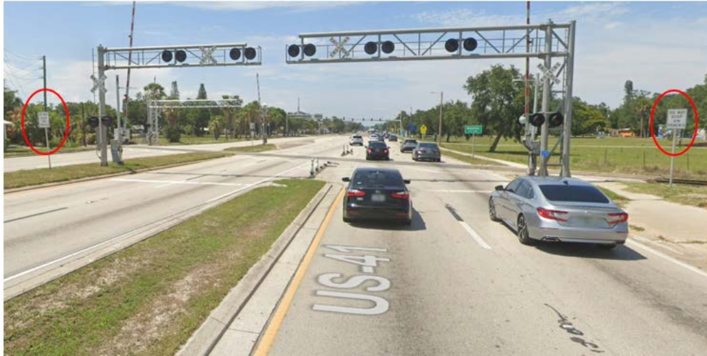
Figure 6-3. R8-8 Signs at US-41 @ 13th Ave E, District 1
