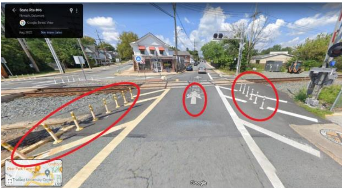
Figure 5-13. Delineators and Pavement Arrows on Westbound at an HRGC in Newark
