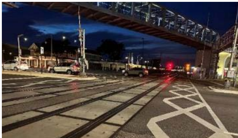
Figure 6-31. Visibility of RDE Pavement Markings at Night at W Colonial Dr @ SunRail Crossing, District 5
