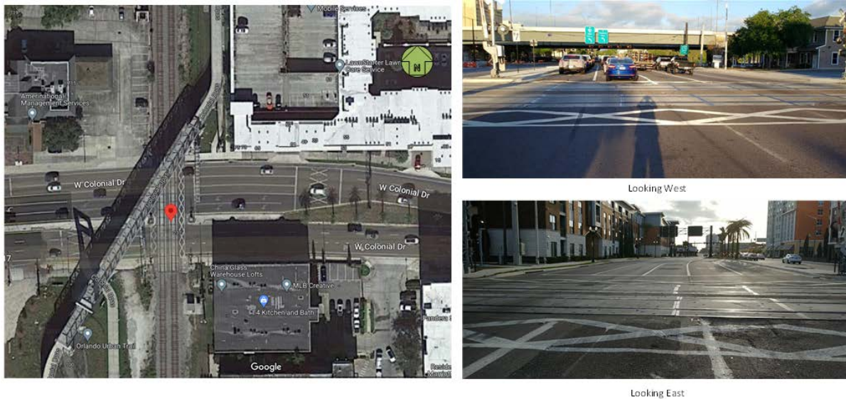
Figure 6-29. Aerial Photograph and RDE Treatment at W Colonial Dr @ SunRail Crossing, District 5
