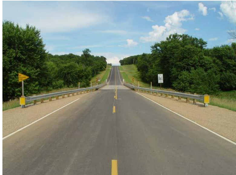
FIGURE 43 Object markers and post-mounted delineators at a narrow bridge.
