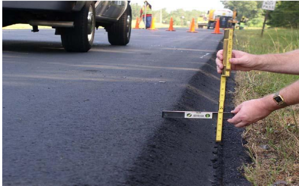
FIGURE 36 Safety edge (top) and after the shoulder has been graded over the edge (bottom).
