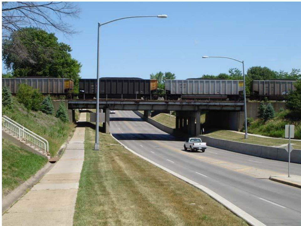
FIGURE 19 Sight distance at an undercrossing.
