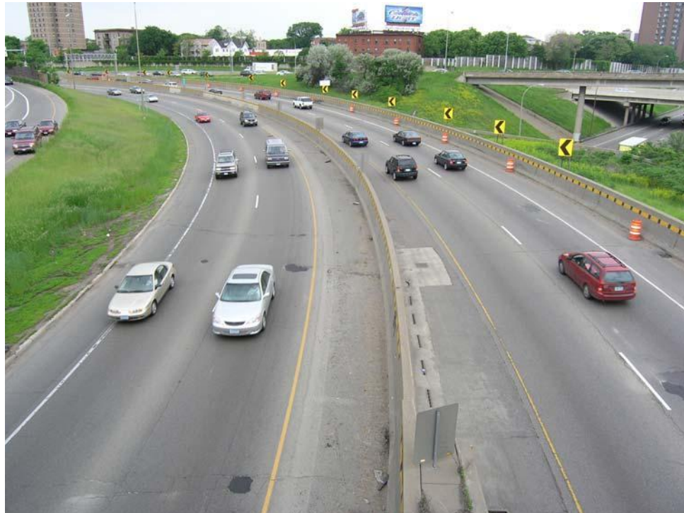
FIGURE 5 Because it is a design control, design speed affects the curvature (radius), stopping sight distance, superelevation, and other features of this horizontal curve.
