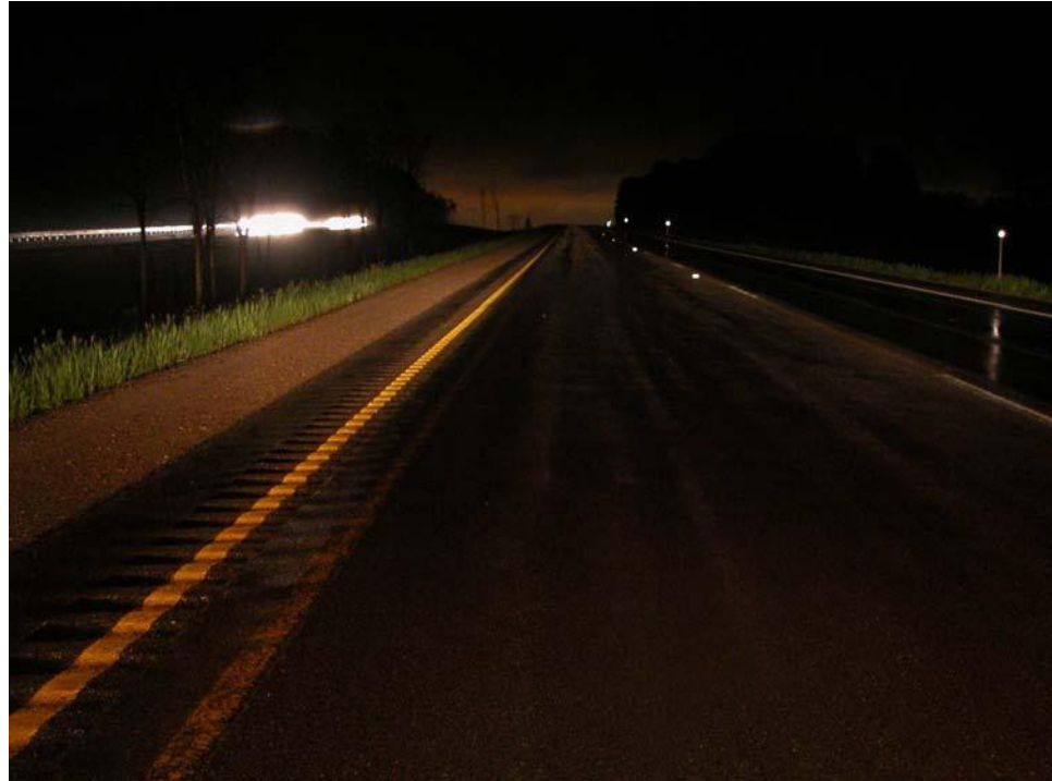
FIGURE 34 Painted edgeline rumble strips.
