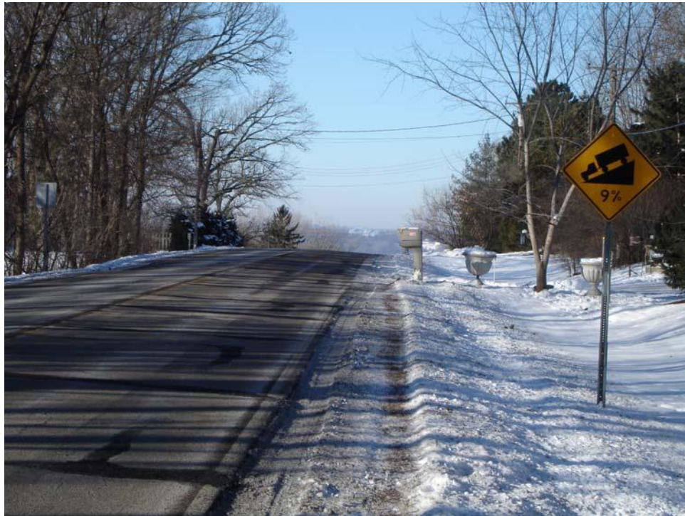
FIGURE 53 Advance warning of a steep grade.
