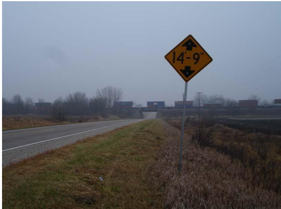
FIGURE 65 Vertical clearance signing.
