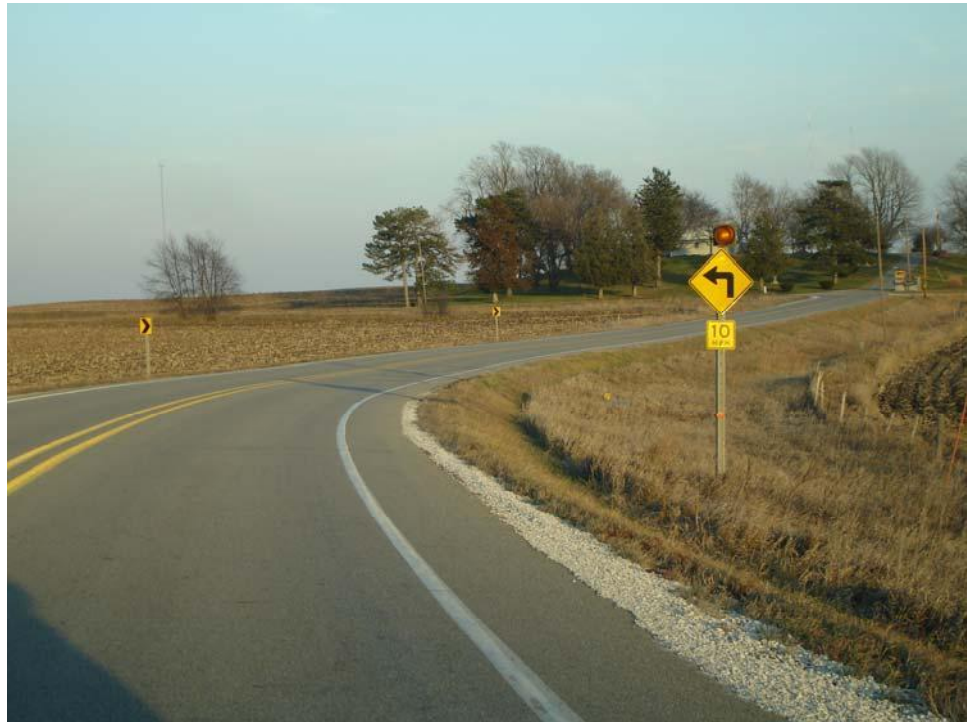
FIGURE 47 Turn warning sign with flashing beacon.
