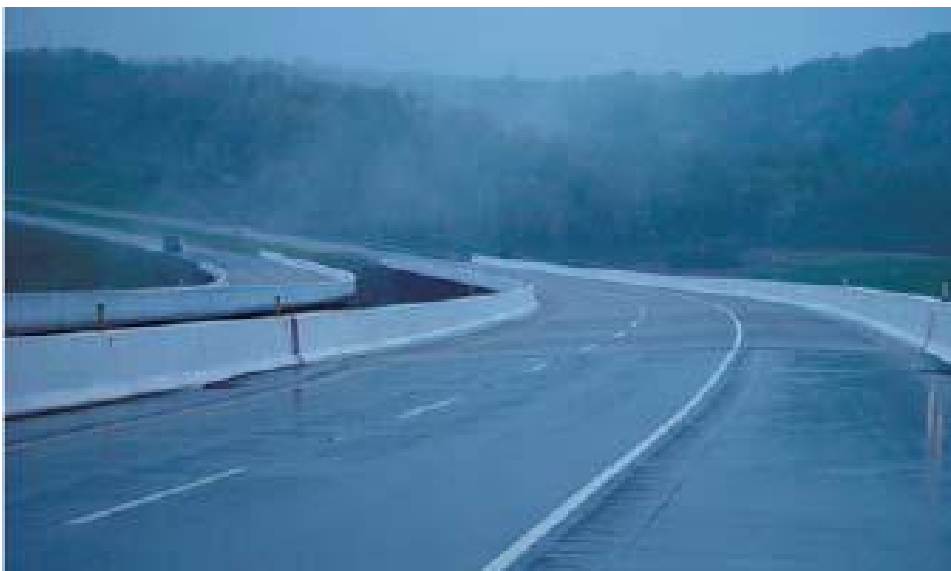
FIGURE 44 White concrete bridge rail.
