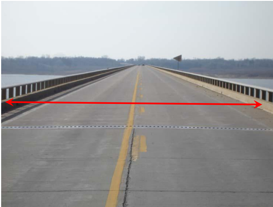
FIGURE 13 Vehicle shying towards the centerline on a narrow bridge.
