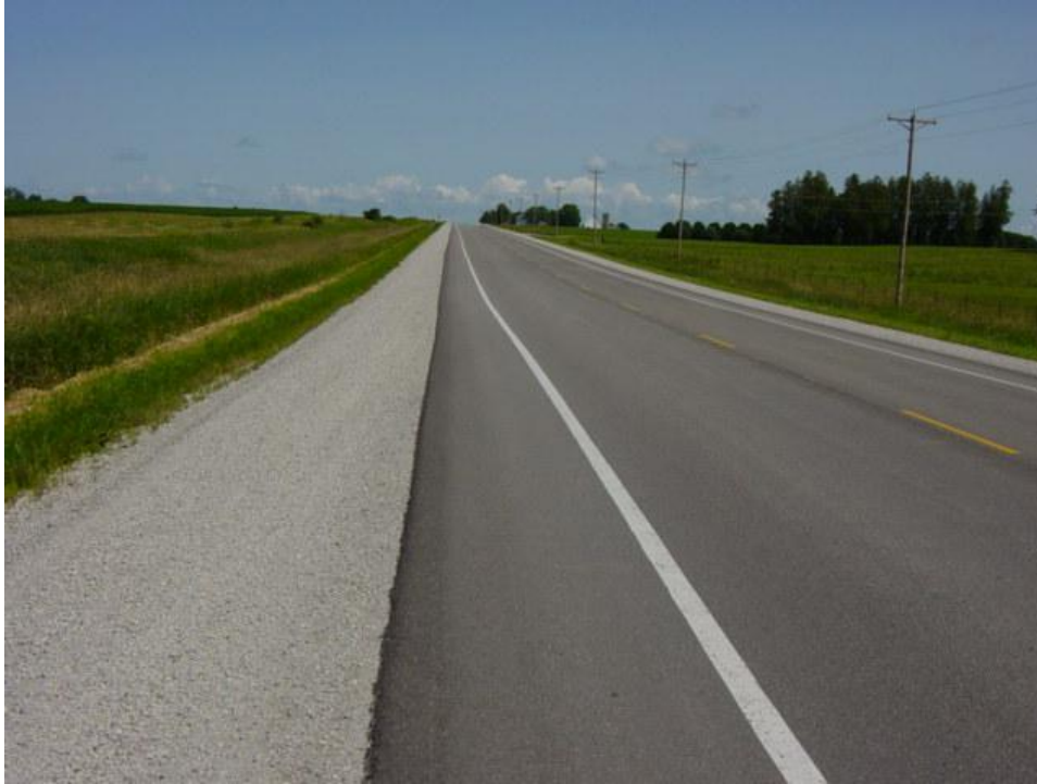
FIGURE 35 Partially paved shoulders.
