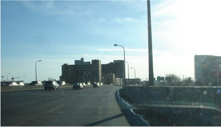
FIGURE 10 Comparison of how shoulder width affects stopping sight distance past concrete bridge rail along horizontal curves.
