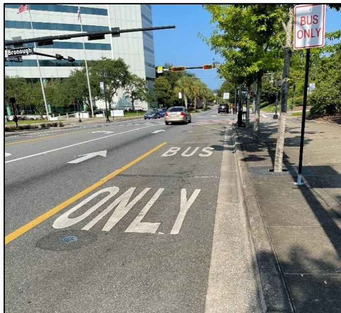
Figure 4.2-1. Pavement Word Markings
