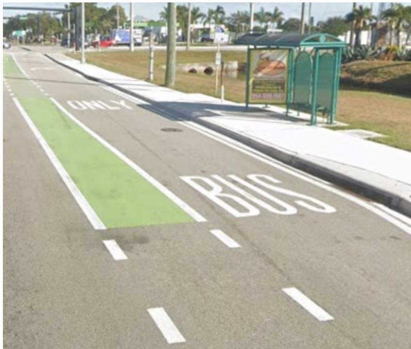
Figure 4.2-1. Pavement Word Markings
